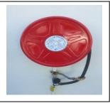
Fire hose reels are used to supplement fire extinguishers. They are designed to be used to extinguish a small wood/paper based fire or to contain a fire while an area is being evacuated. They should not be used on fires involving electricity, cooking fats, or petrol/oil.
