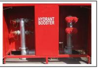
Fire hydrants are used to supply water to the Fire Service if they are fighting a fire on your site. Installation of a fire hydrants are typically require in buildings where there is insufficient coverage from street fire hydrants or where the building area is greater than 500 square metres
