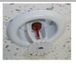
Fire Sprinkler Systems are designed to automatically contain and extinguish a fire. Activated at a set heat/temperature point, fire sprinkler heads automatically operate spraying water over the fire. The activation of the fire sprinkler system typically activates a fire alarm to alert the occupants of the building, as well as notifying the Fire Service.
